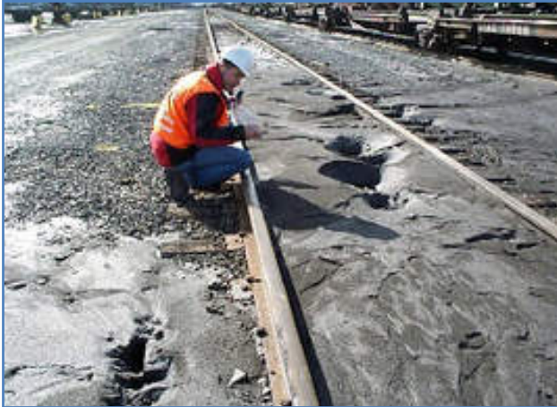
Fig. 3: Sand Boiling
