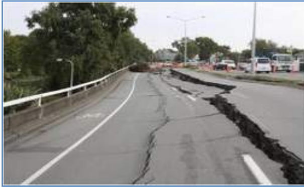
Fig. 4: Lateral Spreading
